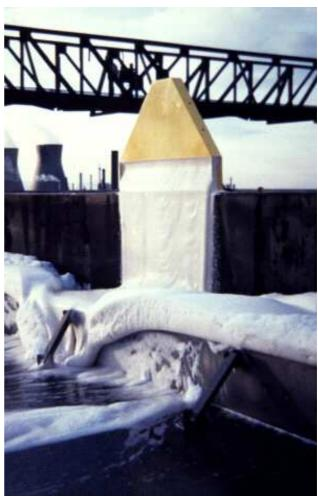
The unit protects the finished foam from wind effects. The aerated fom solution is discharged against the deflector assembly which causes the foam to slide gently down the tank wall into the seal area.
